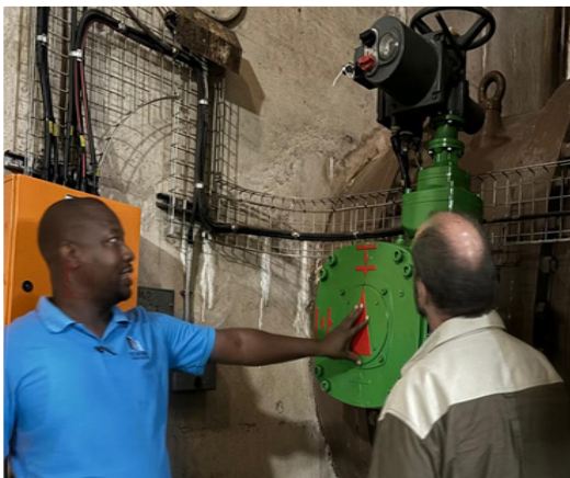
Assistant Water Bailiff, Mr. Vusi Magagula explaining how the Driekoppies Dam valves are operated.
