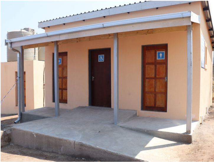
Little Royal Pre-School completed ablution facilities.
