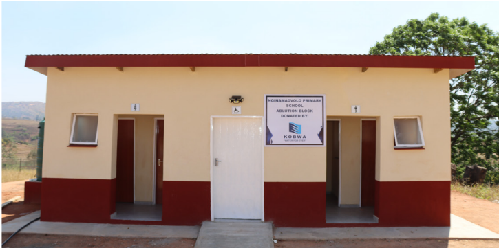
Nginamadvolo Primary School completed ablution facilities.
